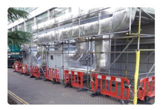
Nominal heating duty 90kW Nominal cooling duty 90kW Air flow (max) 15000 m<sup>3</sup>/h Typical cooled area 2000 m<sup>3</sup> Power supply 415 V 3 ph N+E RUN 84A Noise level (max) 72.2 dBA @ 3m Weight (kg) 1640 kg Plug type BS4343 125 A 5 Pin Average power consumption 26.1 kW/h Duct lenth (max) 48m Duct diameter size 600mm Condensate Gravity drain Dimensions 2280 x 2030 x 2450 Duct size (supply air) 2 x 600 mm Duct sizen (return air) 2 x 600 mm Control Automatic thermostat
