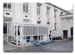
Nominal cooling duty 375 kW 1,279,500 btu Control Automatic programmer Power supply 415 V 3 ph +E 50 hz Run 199 A Plug type Hard wired Noise level (max) 70 dBA @ 10 metres Average power consumption 99 kW/hr Weight 4,800 kg Generator size 200 kVA dependent on system resistance and pump size Dimension 6,058 x 2 438 x 2 591 mm Water connection 4" Bauer
