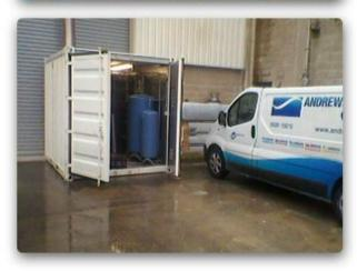
Power supply 230 V 1 ph N+E 50 Hz Run 8 A Noise level (max) 45 dBA @ 10 metres Weight 980 kg Dimension 2,030 x 1,310 x 1,780 mm Fuel consumption 12.5 ltrs/hr Fuel type Gas Oil Plug type BS4343 16 A
